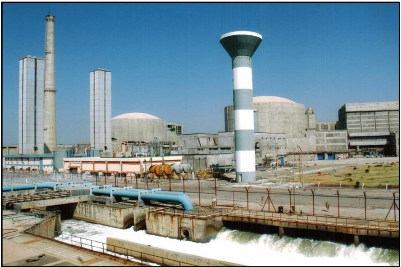
Tarapur Atomic Power Station, (MH) TAPS
